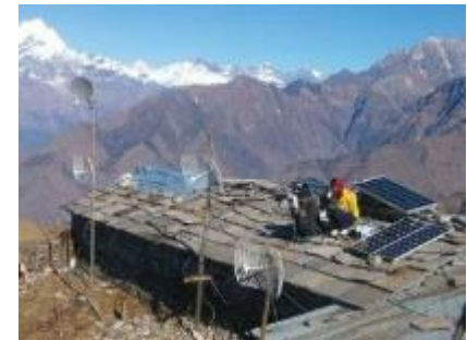
Wireless station in Nangi, Nepal
